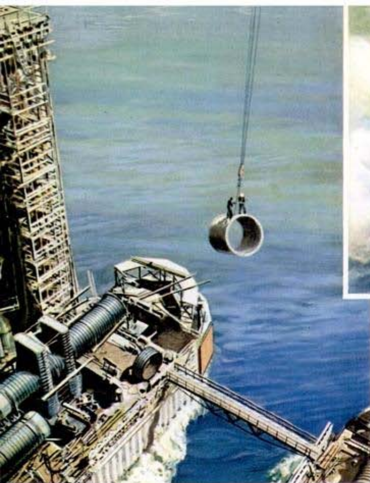
20 A section of outlet conduit is moved into its place
